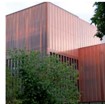
Landeskirchliches Archiv, Nuremberg Exterior walls made of matt shimmering copper with a fine, vertical structure
