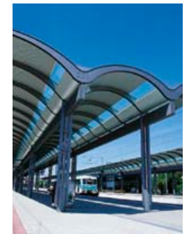
Station platform roofs, type GMP-1
