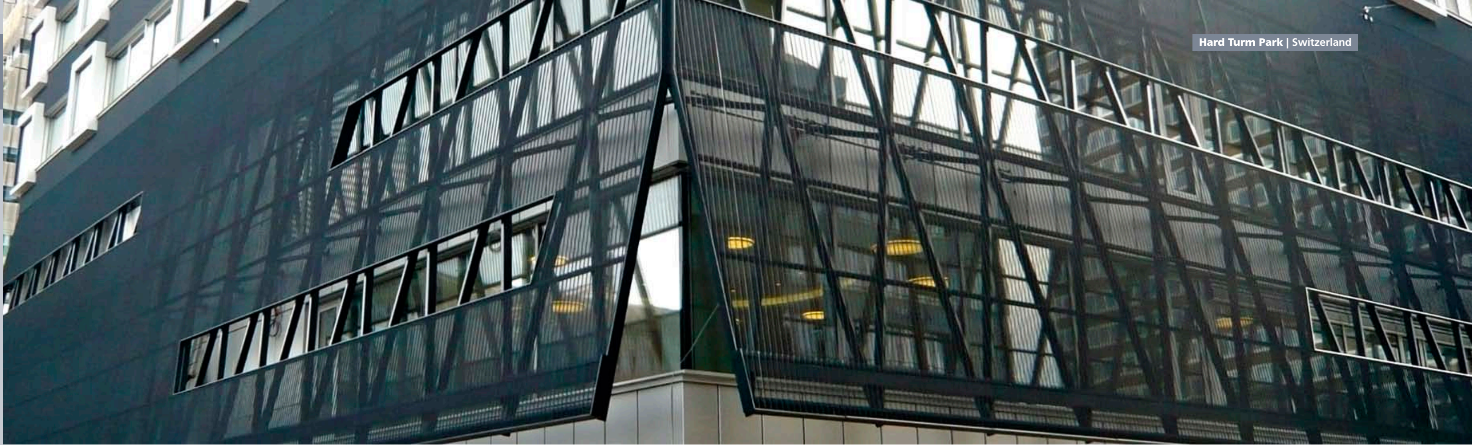
Profile SZ-30/60 R75, (thickness: 1.5 mm), Aluminium, perforated, RV3-4 and unperforated The so-called Röckli (skirting) also serves as a sun shade
