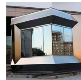
Kulneva, Moscow The 2,000 mm-wide basic material was dyed half in champagne, half in black using a multi-spectral process. It was then edged and relief-milled in one piece in order to obtain as low an edge radius as possible.
