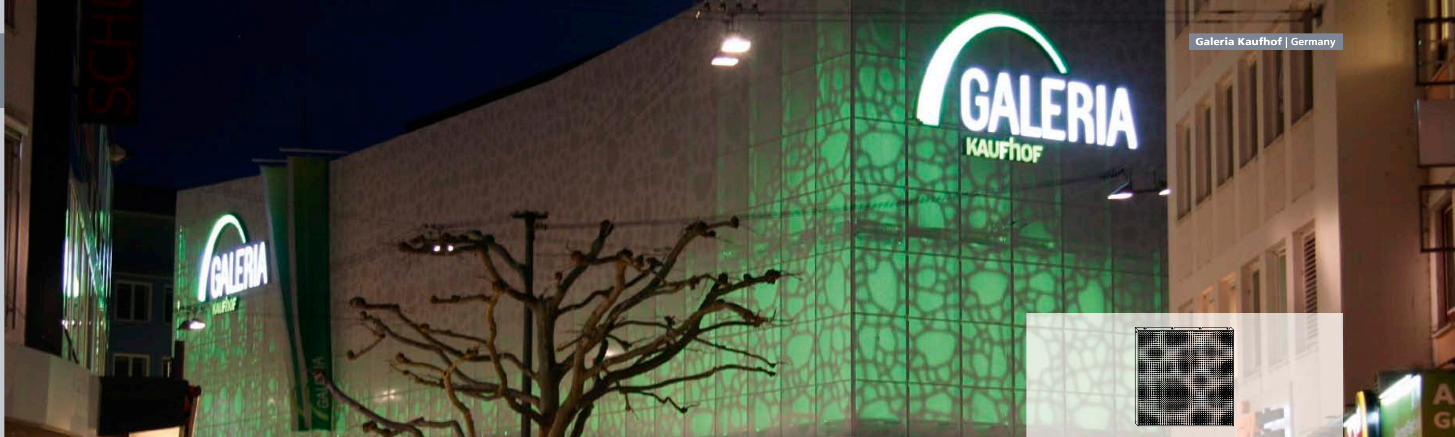
planTEC® system cassette, AlMg3, perforated (Dimensions: 1,510 × 1,510 mm, thickness: 4 mm)
